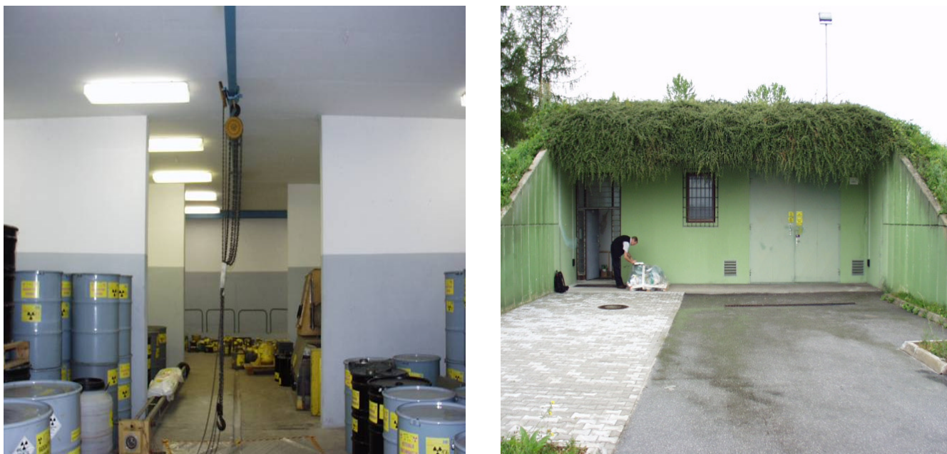
Figure 1: Central Interim Storage for small producers – inside and the front side.
