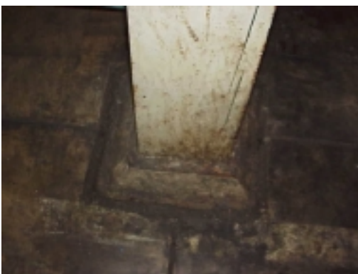
Picture 1: Expansion joints around pillars and between slabs
