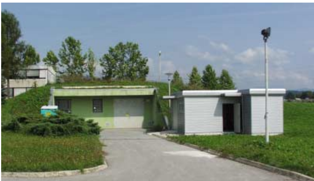
Figure 1: The Central Interim Storage and the newly erected auxiliary building.
