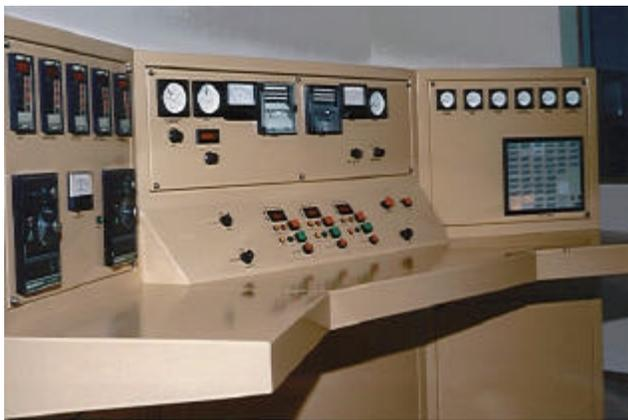
Figure 4. The IPR-R1 Reactor New Control Console
