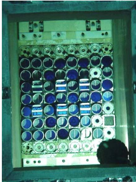
**Fig. 4. HFR core loading pattern at the start of cycle 2003-05**
