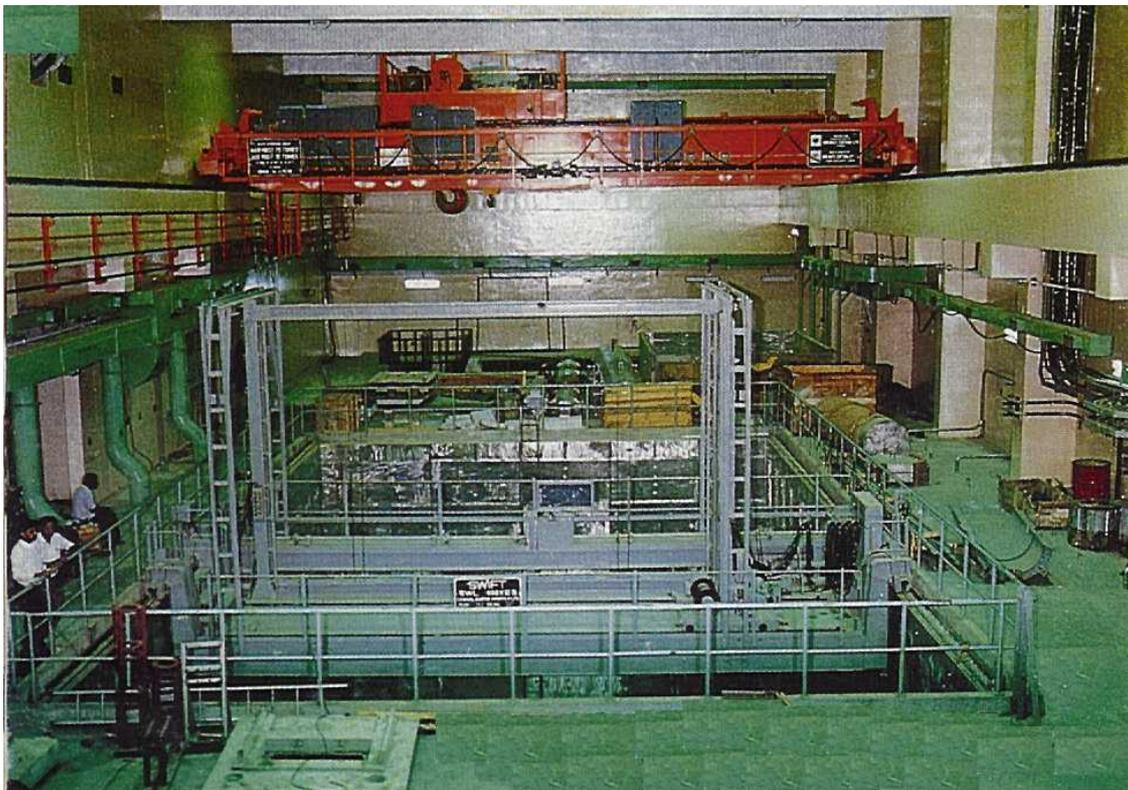
Fig. 3. Spent Fuel Storage Pool at Reprocessing Facility
