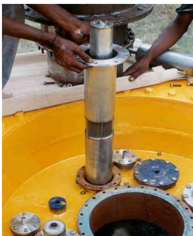
Fig. 9 Removal of tested IHX
