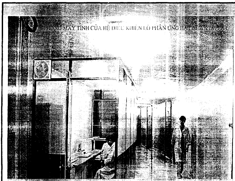
Figure 1: The computer room of the Reactor Control System
