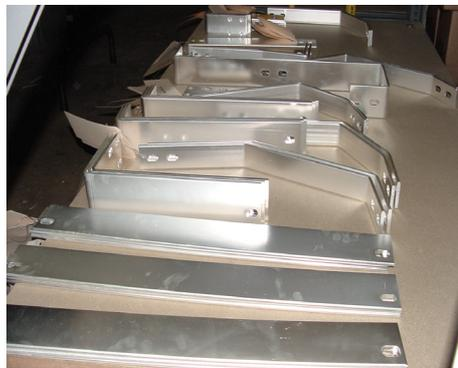
Figure 4: The above picture shows silver plated parts used for metal clad switchgear maintenance.
