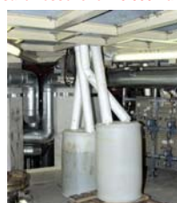
vinyl hoses to drain water from the bottom parts of the machine
