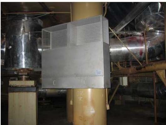
To control the hydrogen concentration inside the containment 15 hydrogen Passive Autocatalytic Recombiners (PAR) are installed in different locations of three different elevation of the containment structure. To allow the required conditions for their operation the FVS controller operates specially installed system for delivering of additional air to the containment with the purpose of assurance of the oxygen concentration needed for effective recombination of the generated hydrogen.
