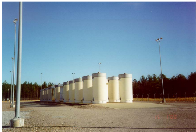
Fig. 3.6.1 DCI casks in service at Surry, USA
