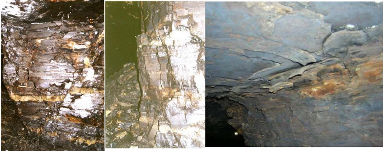
Figure 4: Some fracturing, crack opening in pillars and flaking of roof layers
