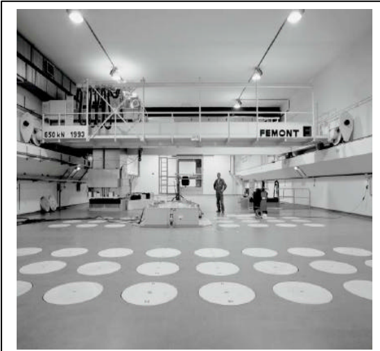
figure 2: Storage building 136 for COGEMA's vitrified High Level Liquid Wastes
