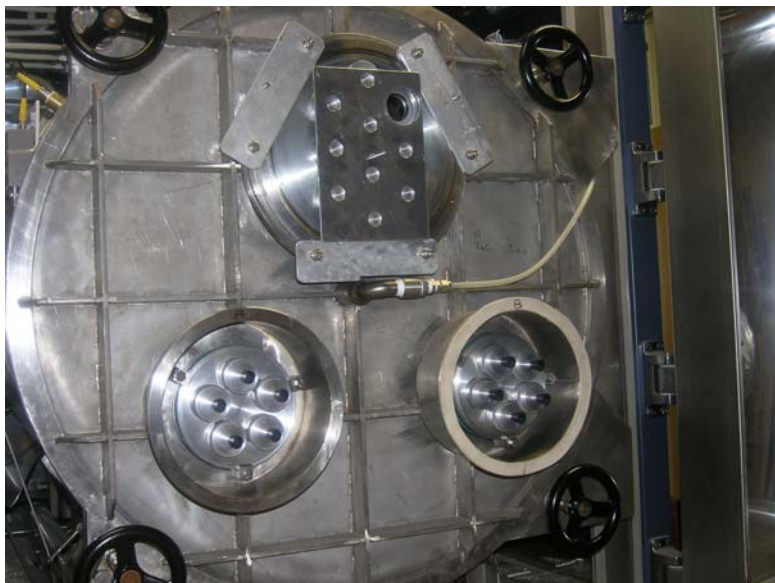
Fig 4 Frontal view of the INMRI-ENEA Climate Radon Chamber
