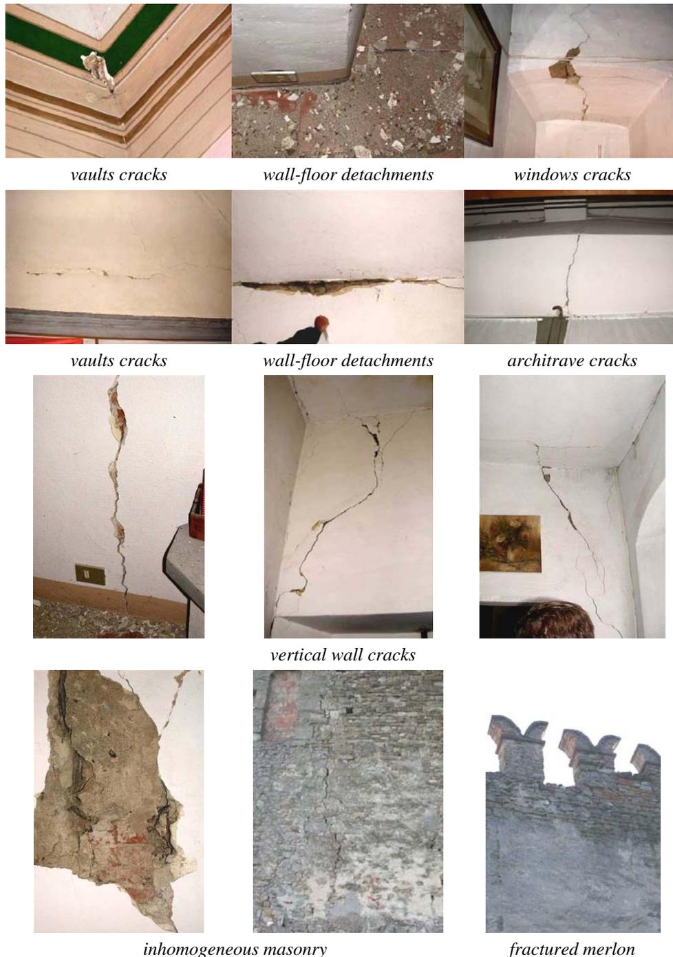
**Figure 13: Principal earthquake damage patterns**
