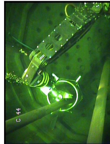
Fig.3 Crushing of a absorber tube
