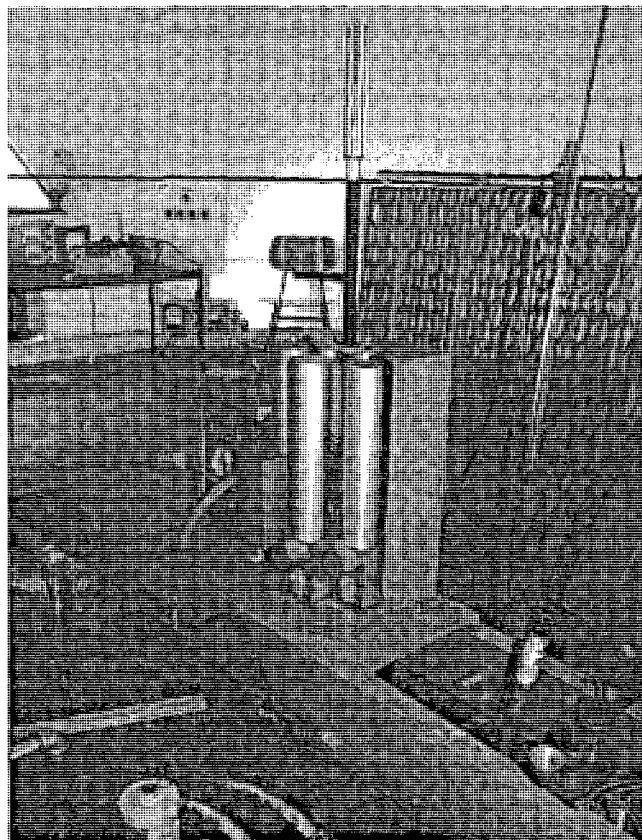
Fig. 4 New control rod mechanisms including a boron carbide pulse rod with compressed air drive (transient rod)
