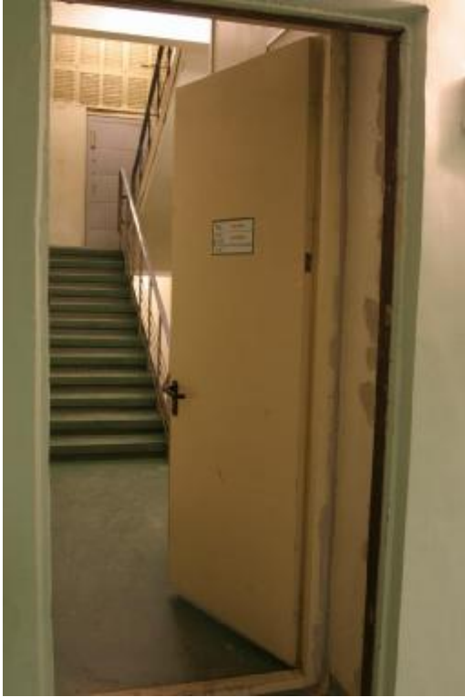
Figure 10 Single-leafed fire protective door
