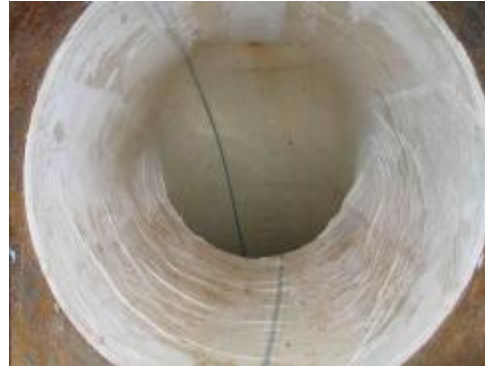
Figure 3 The pipeline after refinement and installation of the anticorrosion coating
