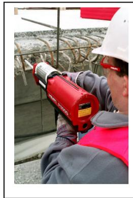
Figure 4: Post-installed rebars
