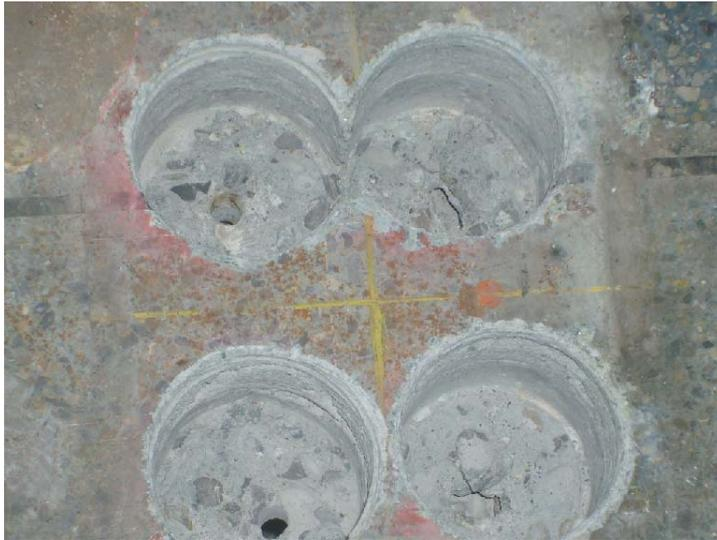
*Figure 10: Extraction of existing screw anchors*
