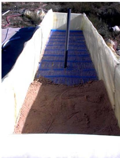
Figure 1: Photo of the solar heat storage unit
