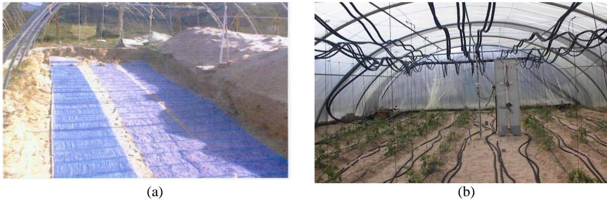
Figure 1. the greenhouse integrated with the designed GHSS: (a) buried capillary plait (b) Agrotherm tubes ringed inside the greenhouse
