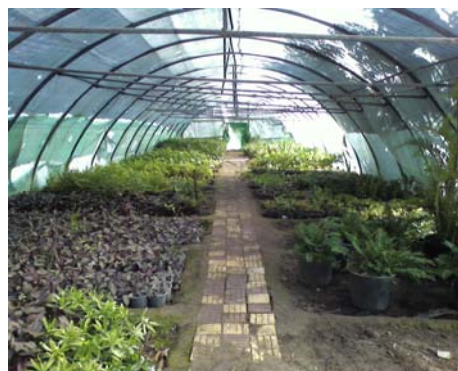
Fig. 2: Photograph for a plastic greenhouse
