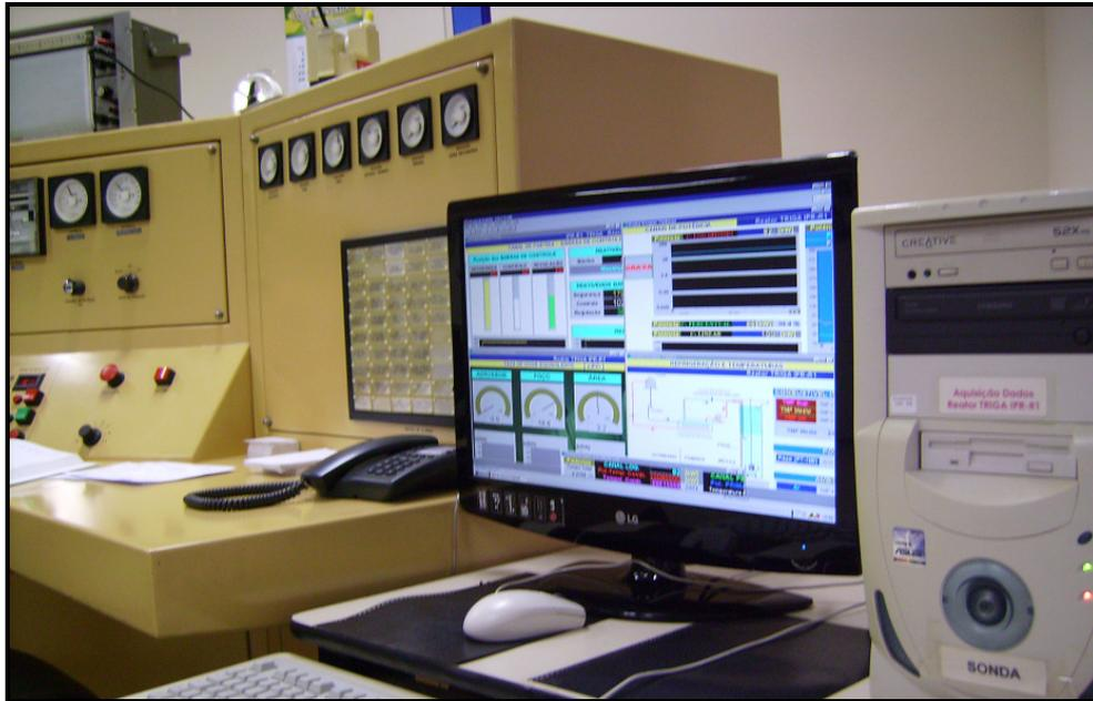
**Figure 2. IPR-R1 TRIGA console and the data acquisition system [4].**
