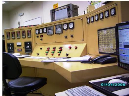
**Figure 3. The first and the current IPR-R1 TRIGA reactor analog control console**
