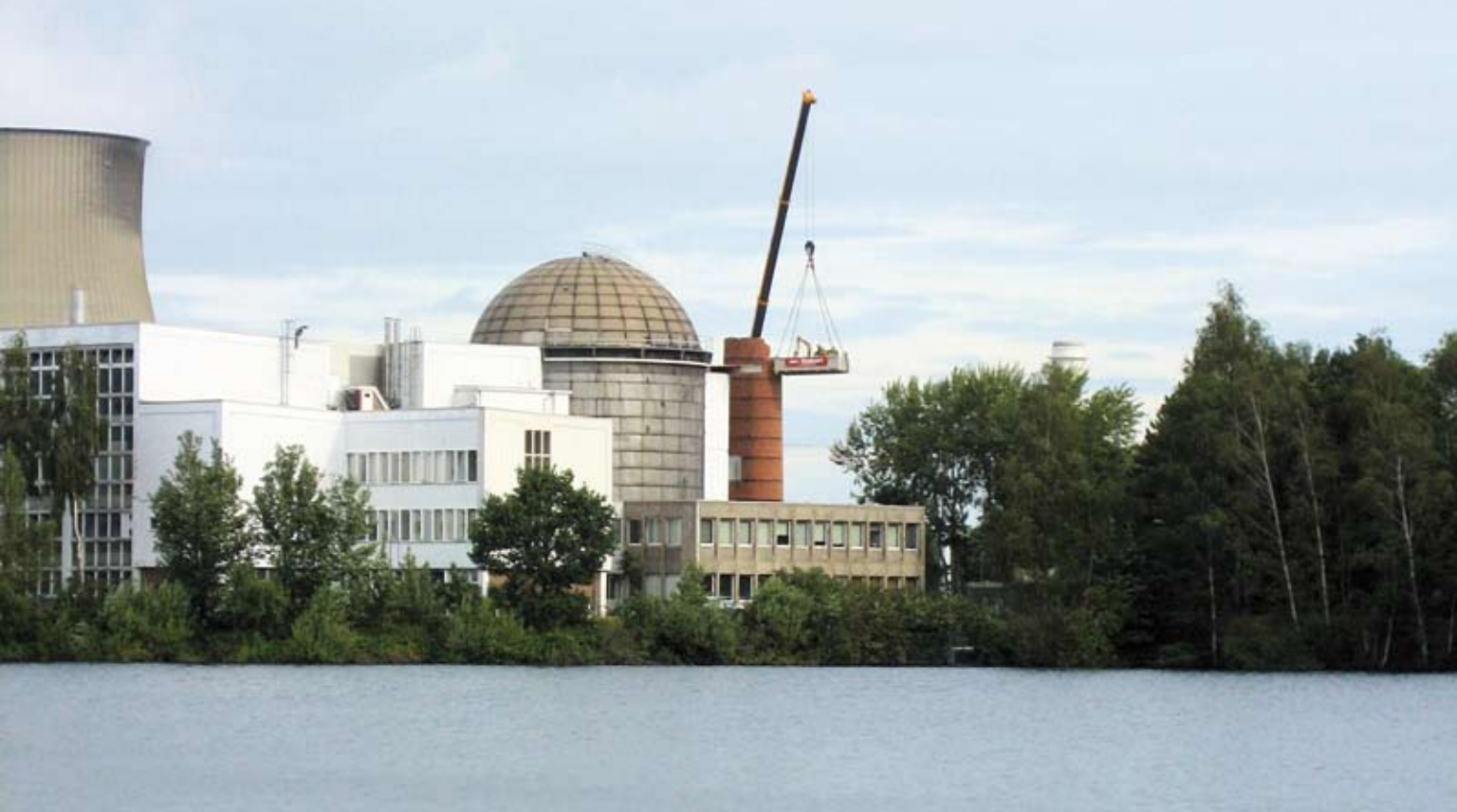
The chimney of the BR3 reactor is dismantled. ↑
