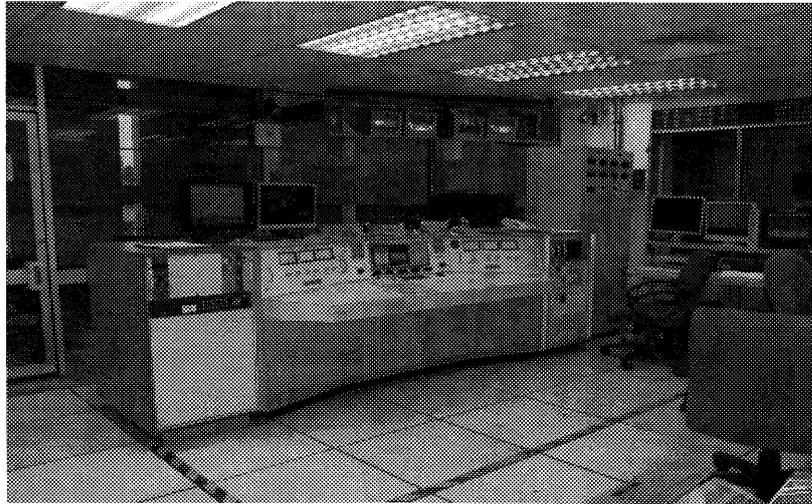
*Figure 1: Analogue Control Console of RTP Research Reactor*
