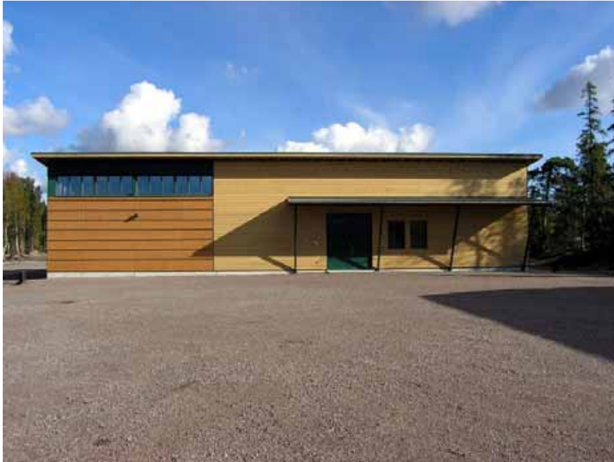
Figure 13. Research building seen from the west (Photo Posiva Oy).
