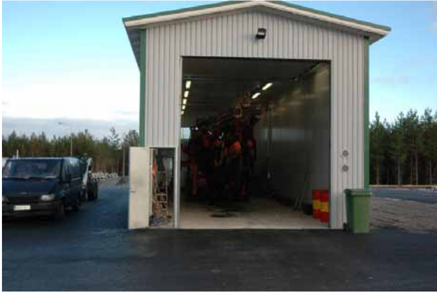
Figure 15. Washing plant to be extended into the repair shop (Photo Posiva Oy).
