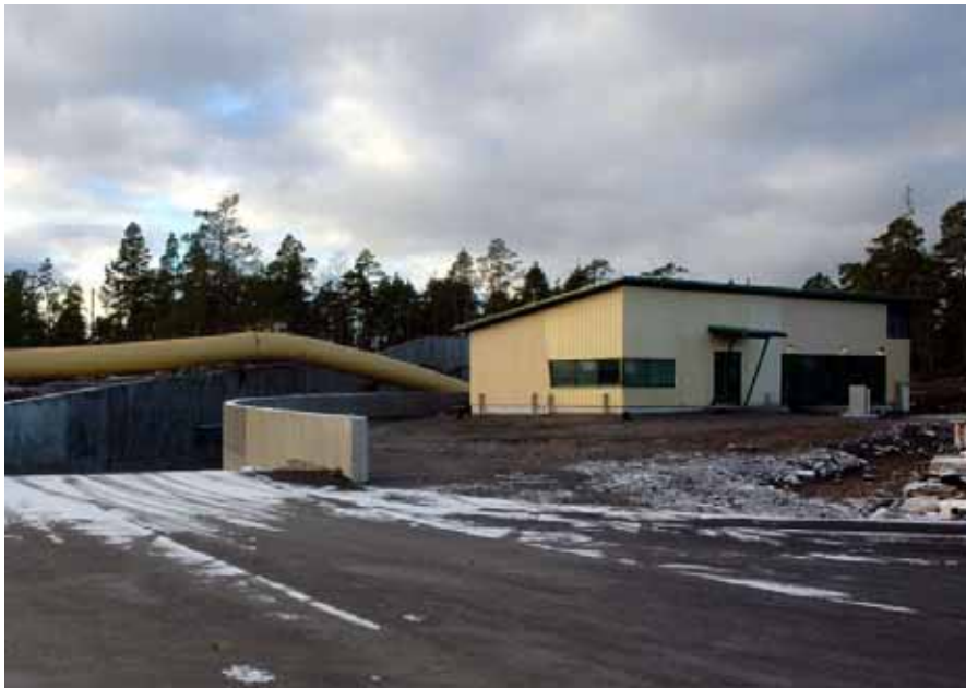
Figure 14. Building for tunnel technology (Photo Posiva Oy).
