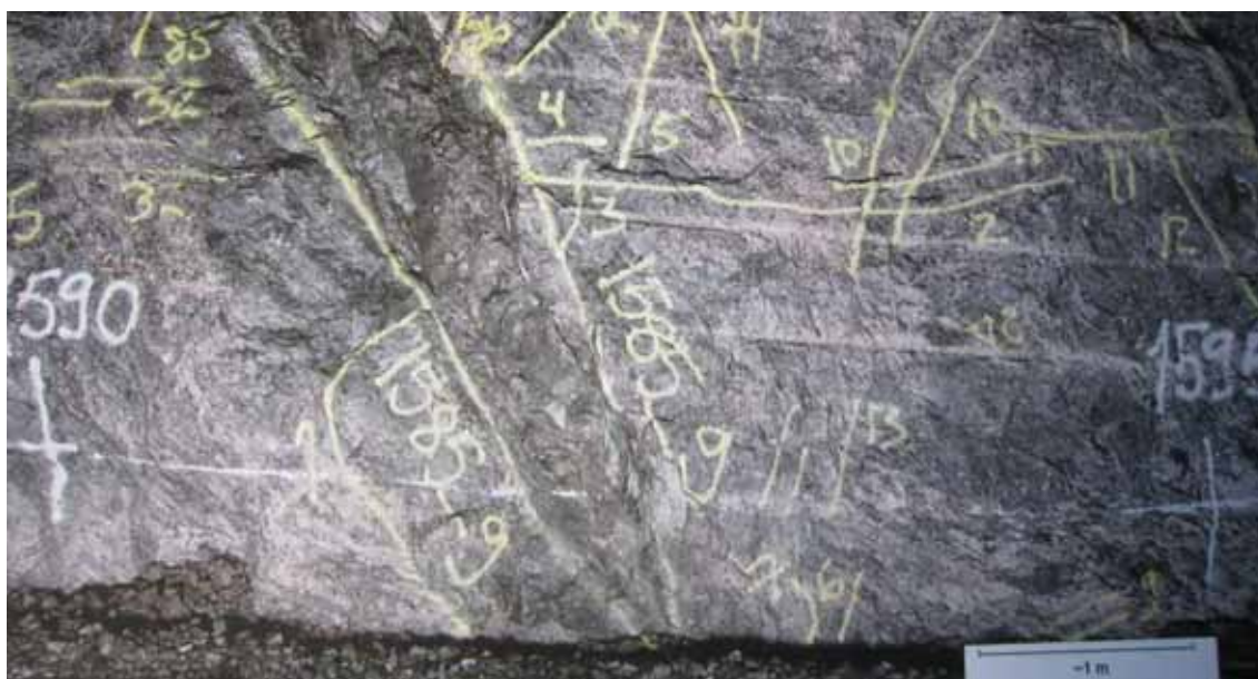
Figure 15. The intersection of fault zone OL-BFZ100 (the "Storage Hall fault") at chainage 1590 m in the ONKALO access tunnel, showing the fault core zone and parts of the damage zones on each side (Photo: Figure 3 in Appendix 6, in Pere 2009).
