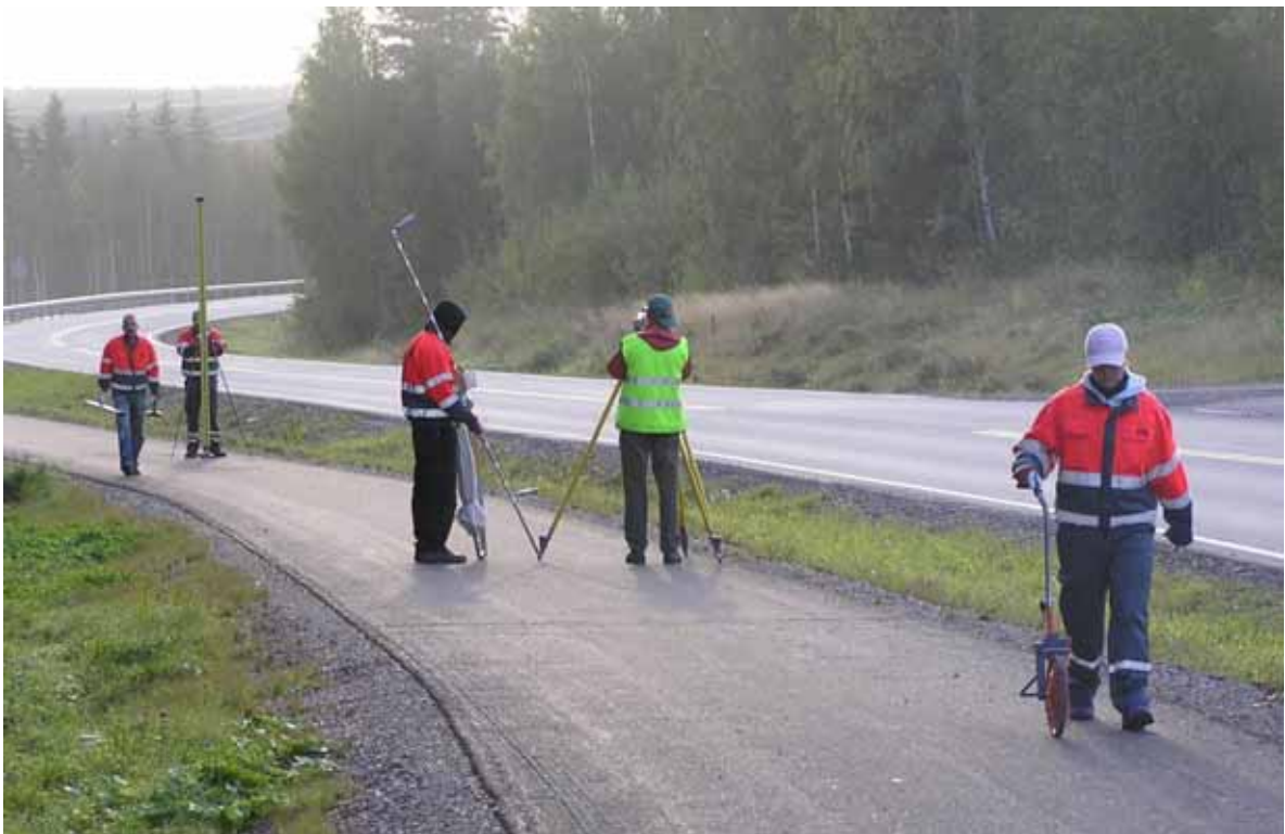
Figure 6. Preparing of the next set up (Photo A. Hiironen) .
