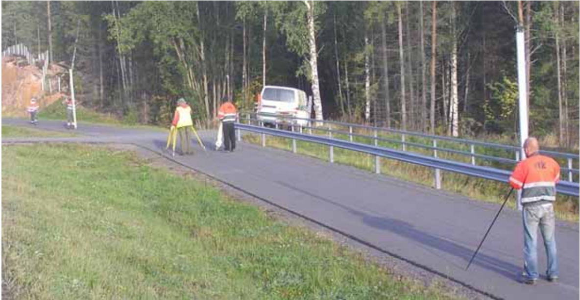
Figure 5. One set up of the bench mark interval 04001-03205 (Photo A. Hiironen) .
