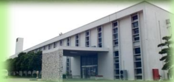
Plutonium Fuel Development Facility "PFDf"
