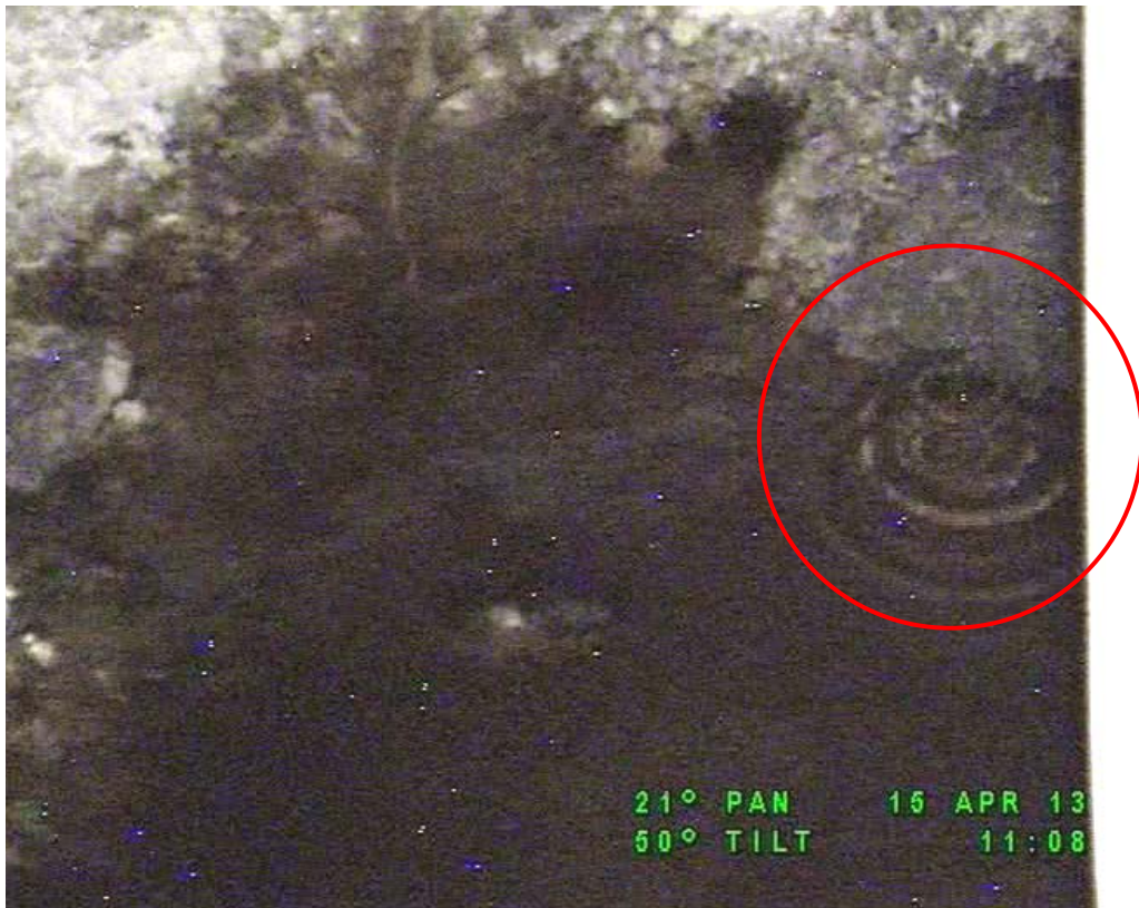
Fig. 4. Tank SX-106 liquid pool ripples.
