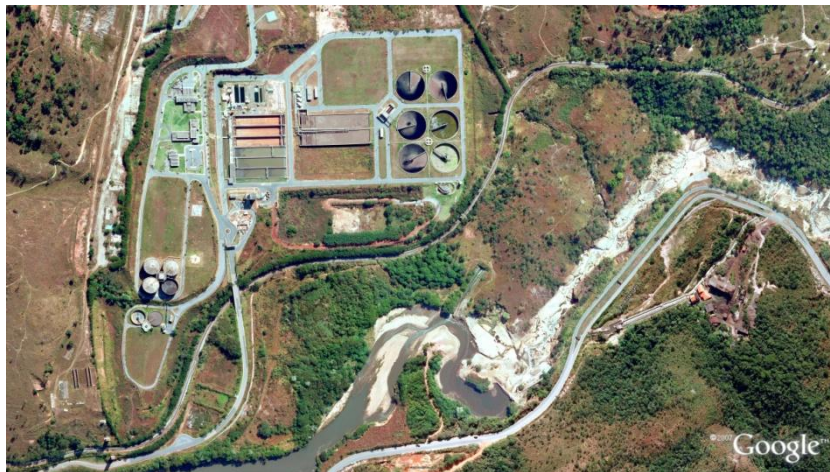
Figure 1. . Aerial photo of Arrudas ETE.
