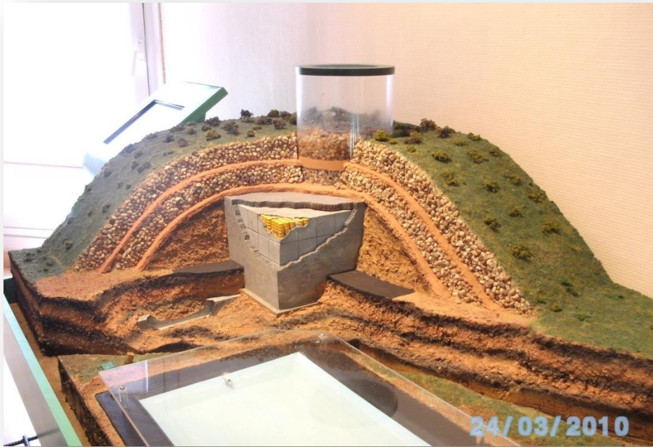
Figure 3: Scheme of the repository – El Cabril, Spain
