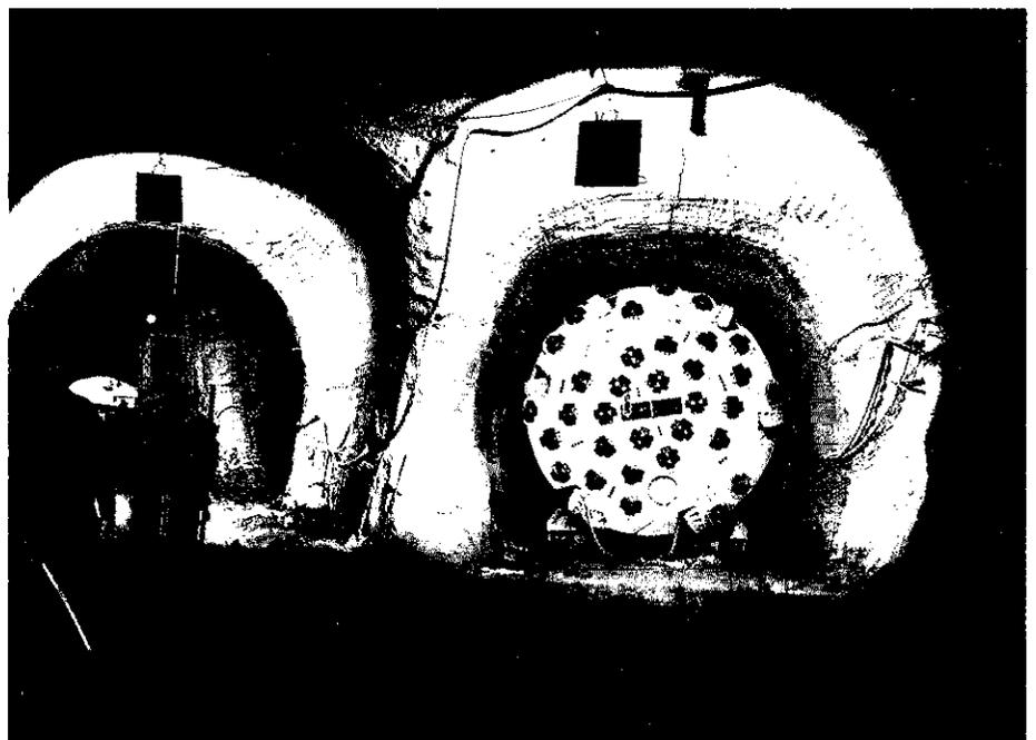
Most of the excavation work for LEP used roadheaders (left) and full-face tunnelling machines (right).
