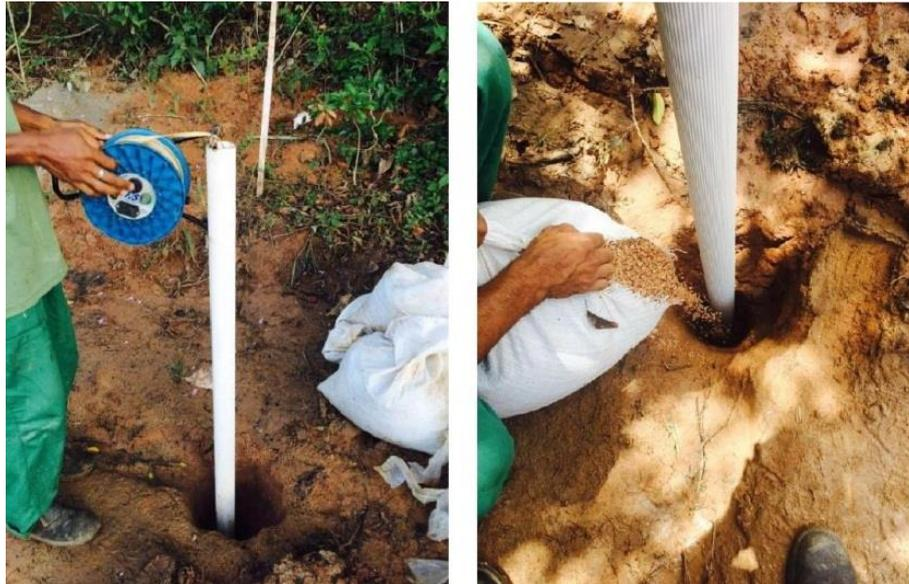
**Figure 7. Construction of a monitoring well**
