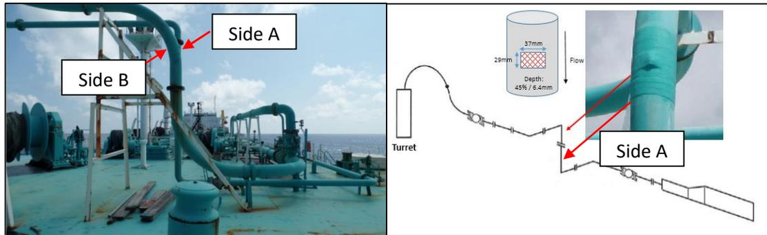
Figure 7: Location of radiographed 10 inch pipe with wrapping
