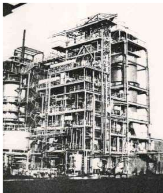
Fig. 5: Photo of Pilot Plant of “Hydrogenating Coal Gasification, HCG”, with a fluidized bed gas generator to convert Lignite, \text{CH}_{0.89}\text{O}_{0.28} , with Hydrogen, \text{H}_2 , into mainly Methane, \text{CH}_4 , at industry site of Rhein-Braun Company, close to the city of Wesseling, near Bonn, south of Cologne. This Pilot Plant was started after the successful operation of a semi-technical plant.
