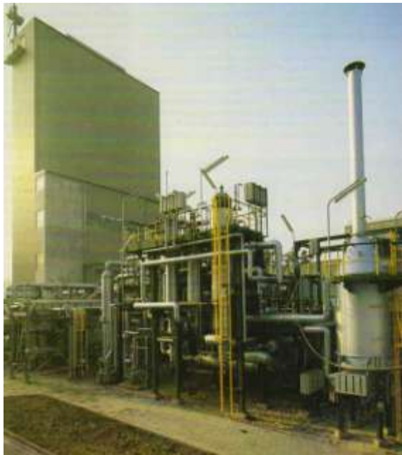
Fig. 3: Photo of Large Scale Test Facility “EVA and ADAM-II”, for semi-technical demonstration of “Helium heated Steam Reformer, REF”, called EVA, as well as for Methane production from Synthesis Gas (H 2 and CO), called ADAM, operated in “Loop Configuration” to simulate the system “Nuclear Long Distance Energy, NLE”, at Research Center Juelich, FZJ, near the city of Juelich, west of Cologne, east of Aachen.
