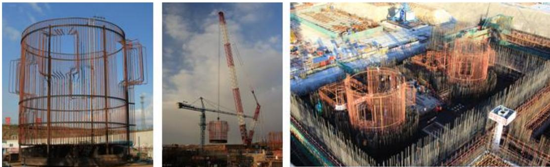
Fig.6 Pre-fabrication and installation of RMA module
