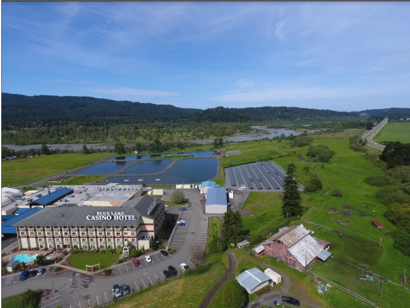
Figure 1- Blue Lake Rancheria site for the MG development
